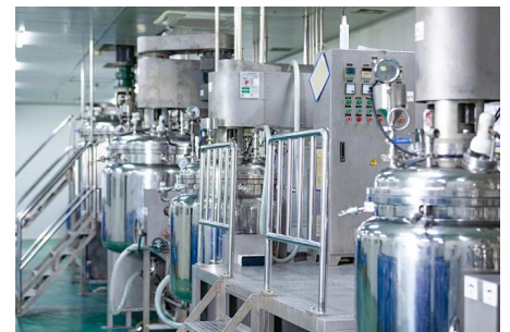
Industrial boiler water degassing
