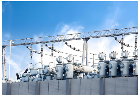
Removal of dissolved gases in power generation
